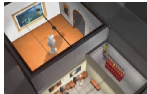
Figure 1: Fixed CO 2 extinguishing system
