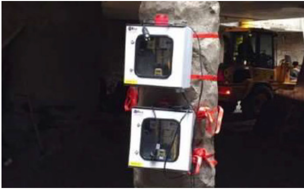
Figure 2: Construction site monitoring with portables.
