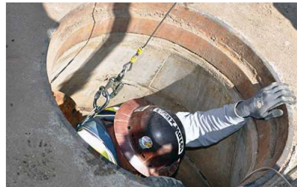
Figure 1. Confined Space Entry
